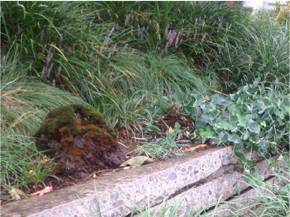
Image 28: retaining wall made of stacked recycled concrete slabs
