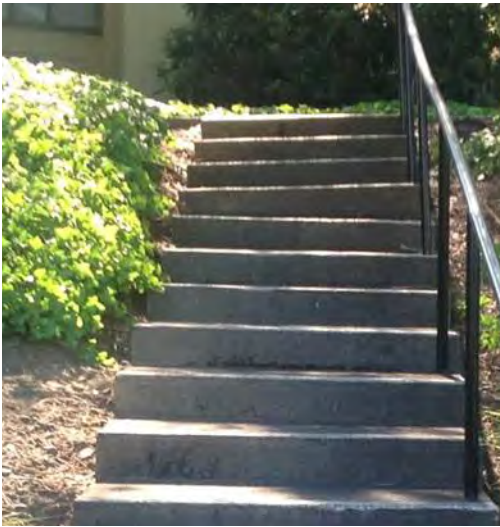
Image 10: Heaving concrete stairs in 2015
